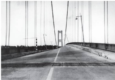
Figure 13.22 The Tacoma Narrows bridge disaster
