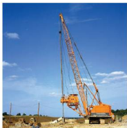
Figure 6.10 When the mass falls, it gains kinetic energy and drives the pile into the ground.
